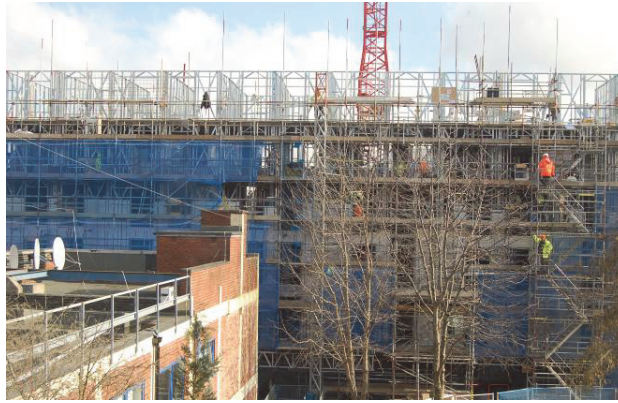
Figure 1: 6-storey building constructed using a cold-formed steel framing system in Sheffield.
