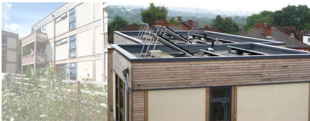
Figure 1. Case study development with PV panels on the roofs (photo MBN).
