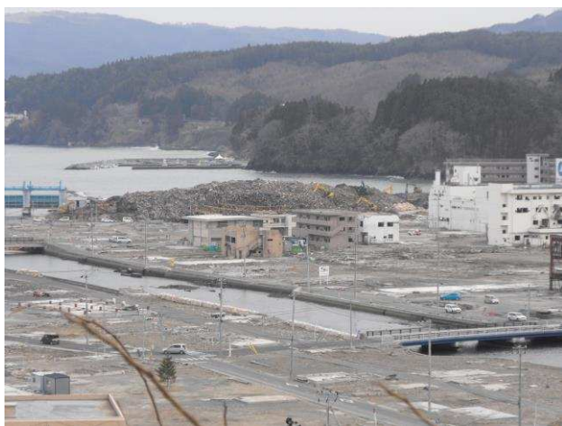
Figure 2: Destruction at Minamisanriku
