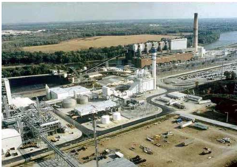
An Coal-to-gas Plant in Indiana
