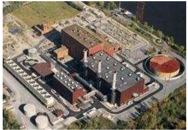
Natural gas plant near Albany, New York. Source: www.pseg.com
