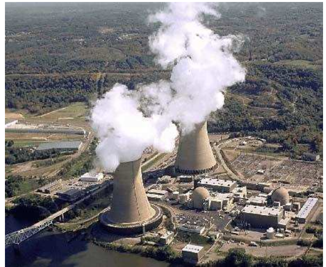
Nuclear plant near Shippingport, PA Source: www.nrc.gov
