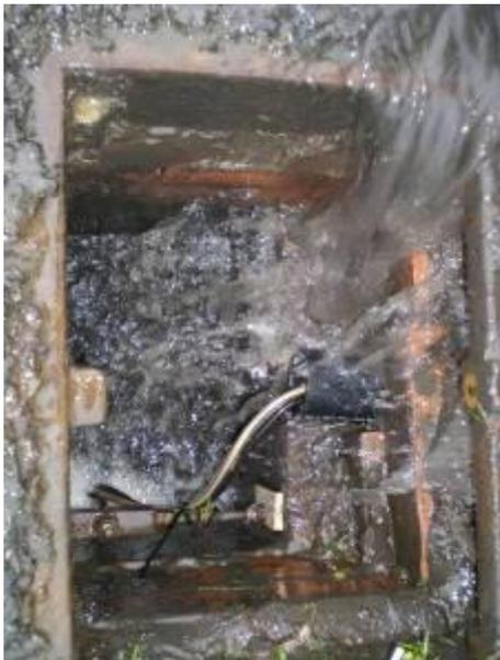
**c) Flow entering gully when grate raised**
