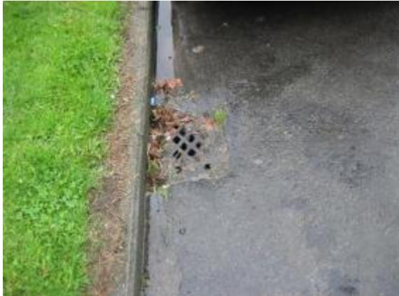
a) A gully grate designed to block (Crichton)
