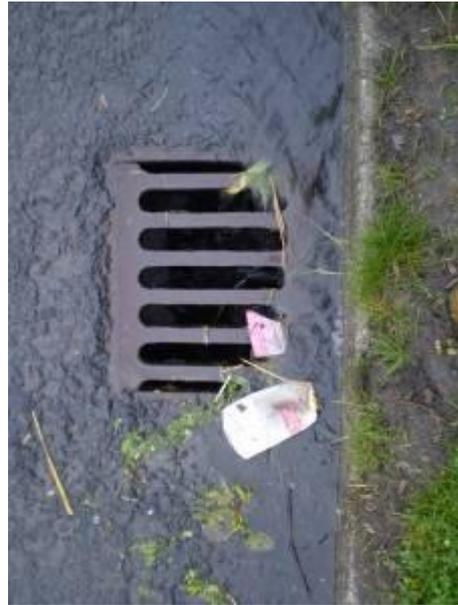
**b) Flow bypassing gully**
