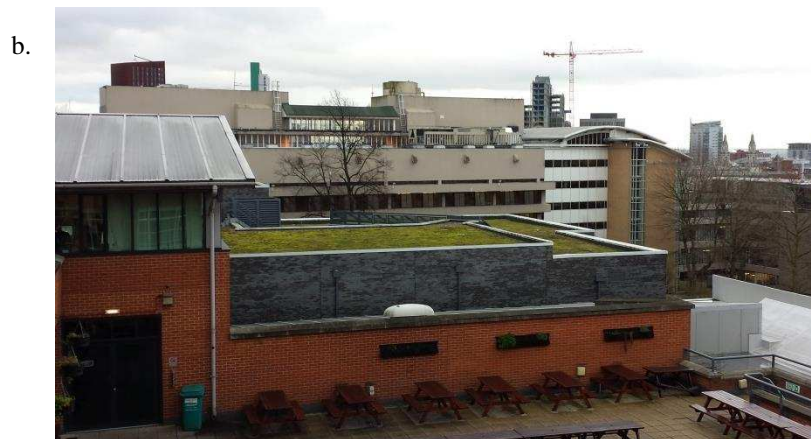
Figure 4.1.1: The extensive green roof above the University of Leeds Performing Arts building in 2007 (a.) and 2014 (b.) (McLaw Living Roofs, 2007).
