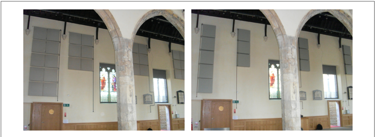
Figure 1. Acoustic panels mounted on the north wall are closed and folded in half (on the right).
