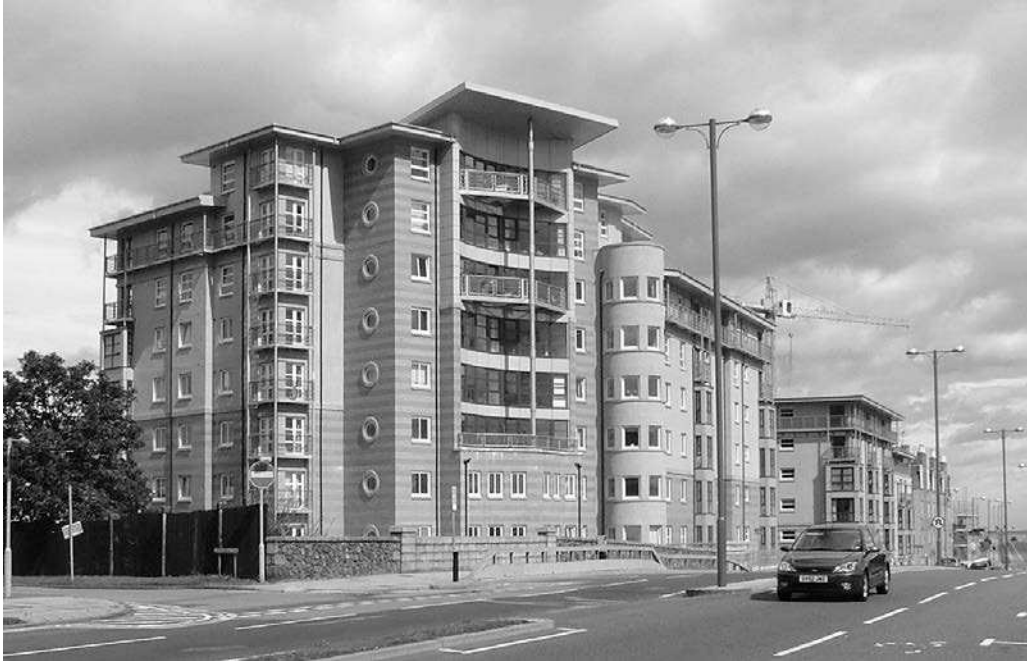
Figure 2 A typical pragmatic bespoke flatted development, Aberdeen, Scotland. Source: Photograph taken by Dr Steven Tiesdell and reproduced with permission from Professor David Adams, University of Glasgow.
