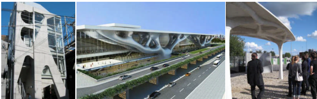
Figure 2 - a) An office building in Japan with topology optimised Walls; b) A topology optimised support structure; c) Topology optimised support structure for a Canopy in Doha
