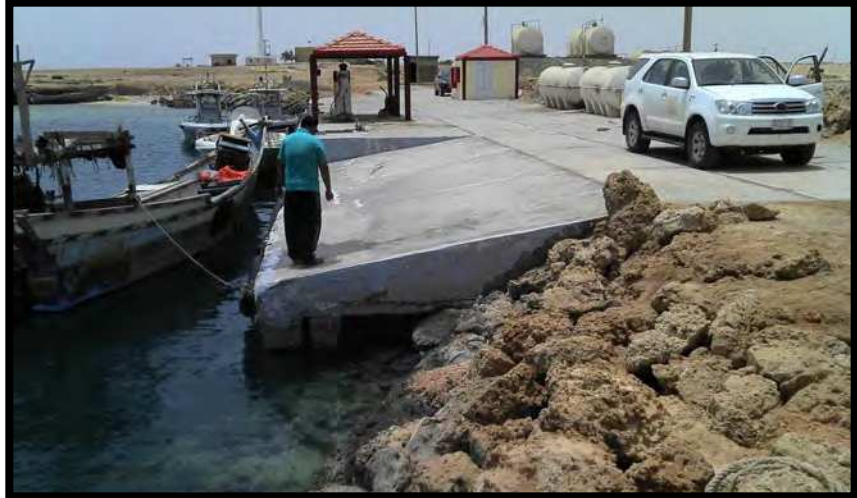
Figure 22: The temperature loggers are located at the foot of the quayside in protected waters, sheltered from both rough weather and fishing boats.
