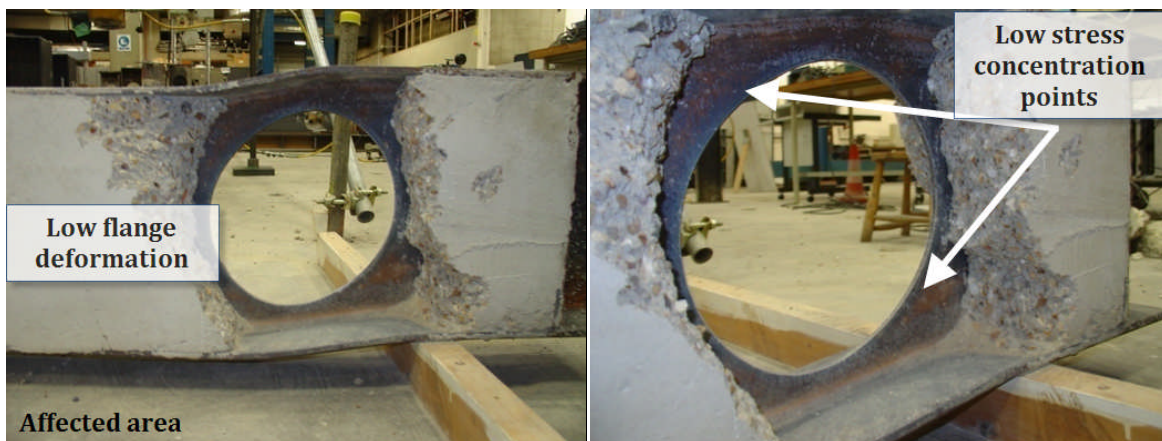
Fig. 17: Failure mode for partially encased USFB No.1 at opening after removal of the damaged concrete
