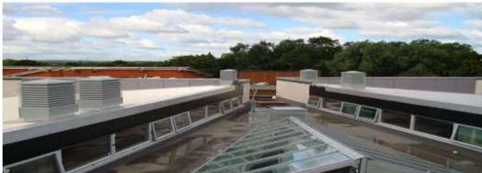
Leicester School building
