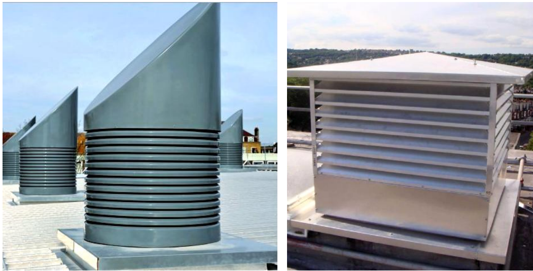
Figure 5 Modern roof mounted circular and square wind tower systems (Hughes et al., 2012)
