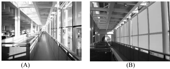
Figure 8. ICoSS south-facing façade shading schemes: (A) No shading is provided; (B) internal roller blinds applied
