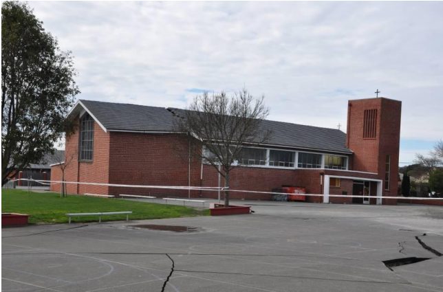
Figure 5.30: St. Paul's church in Dallington area - overall view of building looking north-east.
