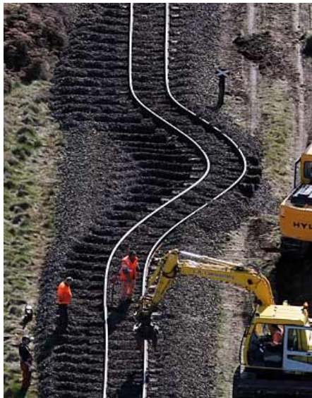
Figure 7.35: Railway Embankment at Rolleston (photo by I. McGregor).
