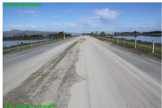
Figure 6.30: Repaired Dyers road that runs between Ponds 2A and 3. ( -43.529933^\circ , 172.715200^\circ ).
