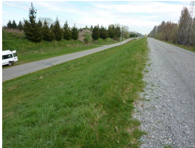
Figure 6.9: Photo 6: Stretch of stopbank without evidence of liquefaction. In the distance, a small rise can be seen in the road. This rise is the start of the ~0.5 km stretch where liquefaction was observed along the base of the stopbank. (43.4225°S, 172.6350°E).
