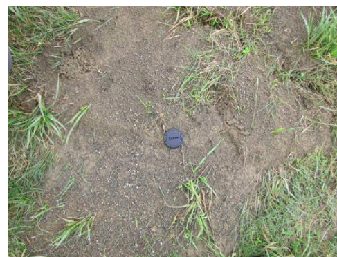
Figure 4.38: Liquefaction on the grass verge adjacent to the end of Gillanders Rd (Darfield side). Note the fine gravel particles on the surface and the fissure towards the top right hand side - it was possible to push the sampling spoon to a depth of about 300 mm into the fissure. (Position marked as Photo 2 in Fig. 4.36).
