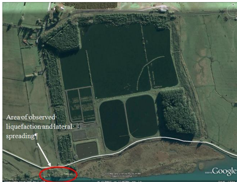
Figure 6.27: Aerial image of the Kaiapoi Sewage Treatment Plant. The southern perimeter (~0.6 km) of the oxidation ponds (bottom of image) forms the stopbanks of the north side of the Waimakariri River. (43.384583°S, 172.688240°E).
