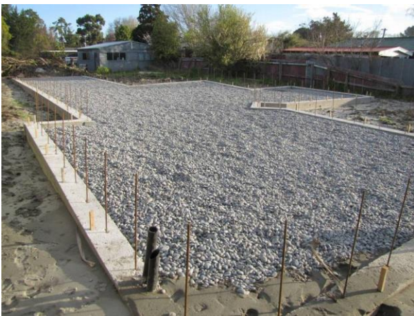
Figure 5.41: Site at Pines Beach which appears to be using the same slab-on-grade system as at Bexley (Chichester Street)
