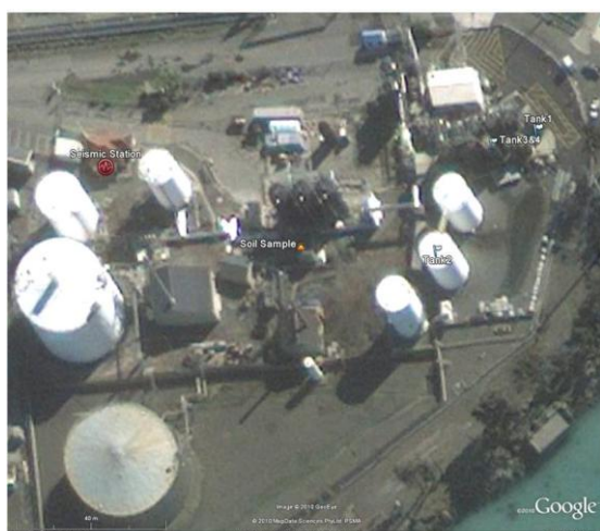
Figure 7.41: Zoomed into the region of the Fulton Hogan Bitumen Plant. (GoogleEarth image; 43.6088°S, 172.7140°E).
