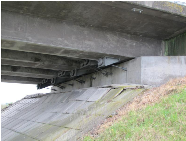
Figure 7.22: Cable Restrainers at north abutment, Chaney's Overpass.
