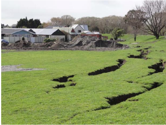
(a) Lateral spread and slumping of the north stopbank of the Kaiapoi River near the east end of Charles St; note the huge piles of cleaned up sand obstructing the view of the houses.
