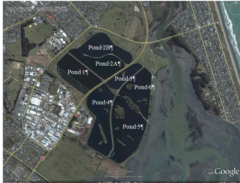
Figure 6.29: Aerial image of the Bromley Sewage Treatment Plant. ( -43.535029^\circ , 172.714052^\circ ).
