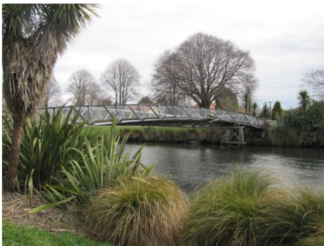
(a) Buckled span.
