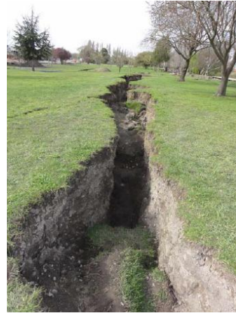
(b) Lateral spreading of the north stopbank of Kaiapoi River (Charles St – Jones St).
