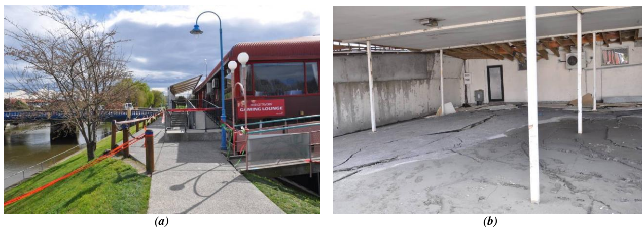
Figure 5.13: Bridge Tavern adjacent to the Kaiapoi River. (a) view looking northwest at Williams Street bridge and (b) view looking northwest at subterranean parking.
