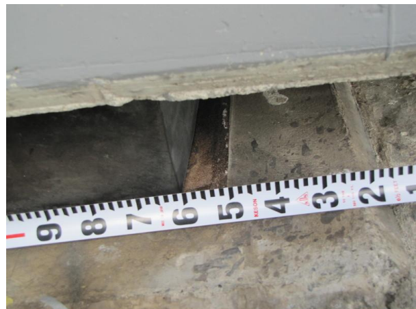
Figure 7.5: West abutment bearing pad displacement, Bridge Street Bridge (scale in Inches).
