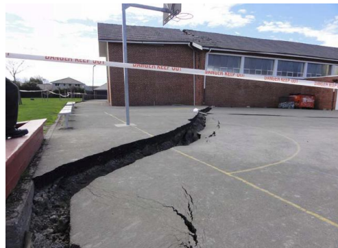
(a) Bearing failure in liquefied soils (St Paul's Church, Dallington); the crack is 500-900 mm wide with a vertical offset of 330 mm, at its maximum.
