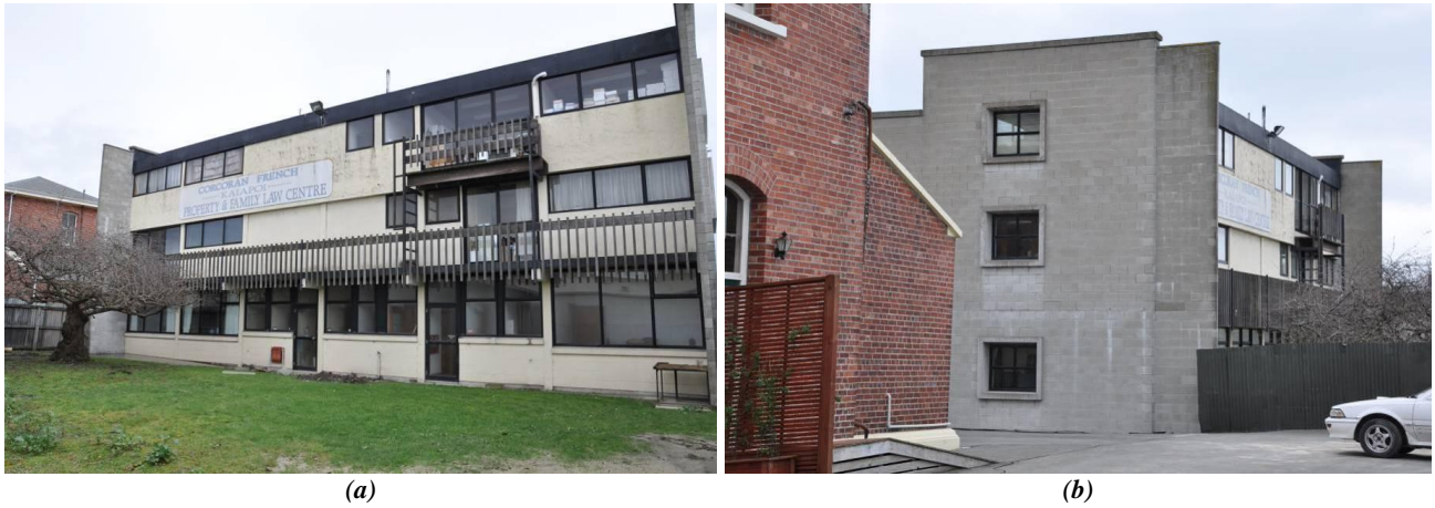
Figure 5.7: Property and Family Law Offices in Kaiapoi business district. (Williams St.) (a) View looking northwest (at long axis end) of building and (b) view looking northeast showing shear wall ends of short axis of building.
