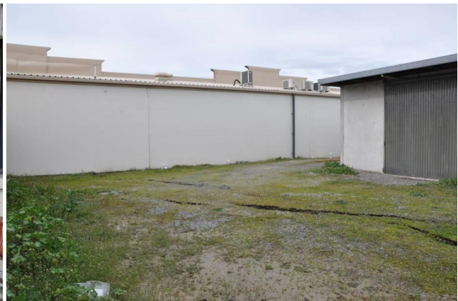
Figure 5.9: Surrounding ground failure patterns directly adjacent to the Property and Family Law Offices in Kaiapoi business district. View looking southeast.
