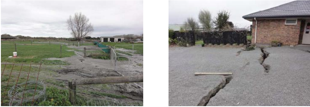
(a) Sand boils and lateral spread cracks.
