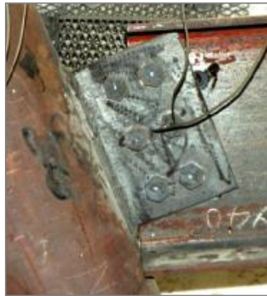
Fig. 11 Failure of the fin plate connections at 550°C.
