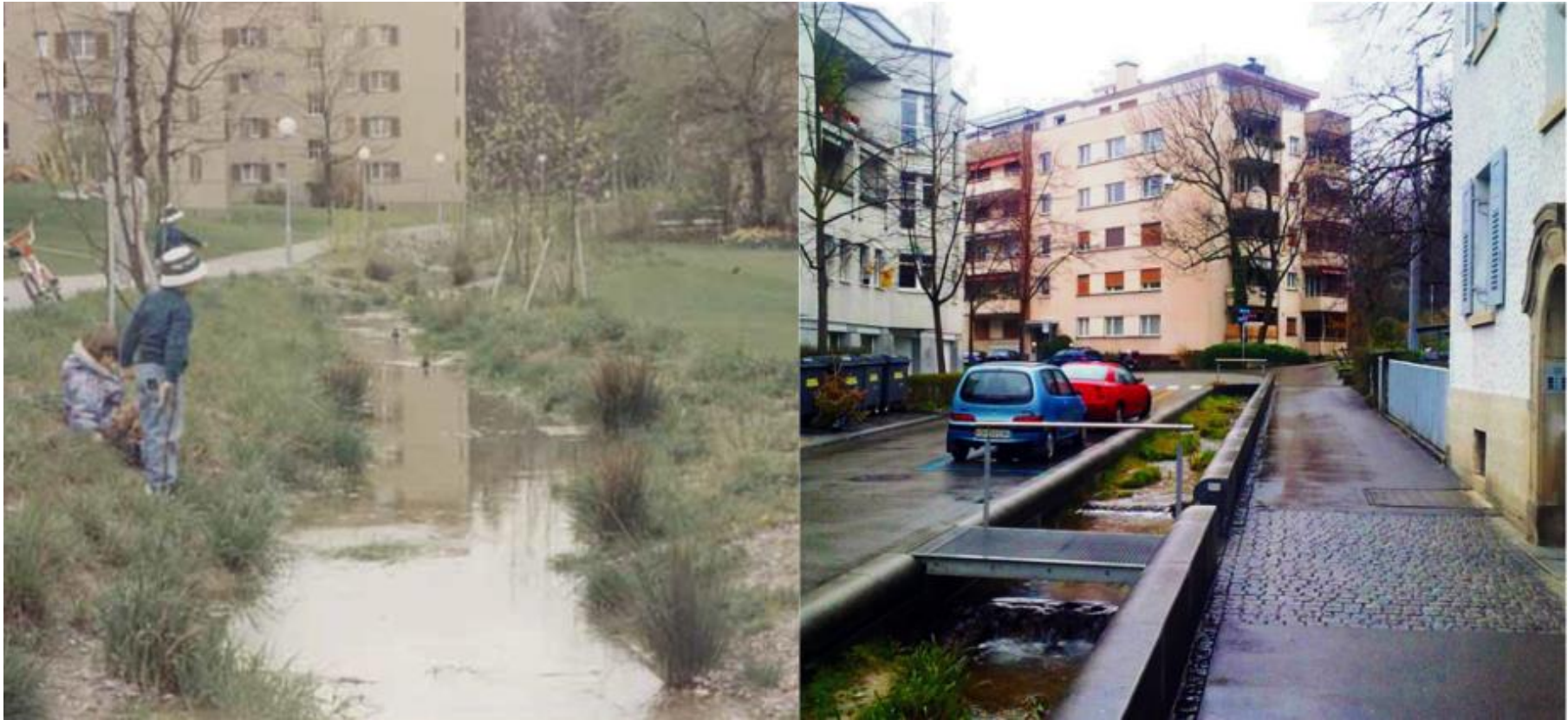
Figure 5 Daylighting urban streams for captured stream and spring separation from combined sewers: the experiences of the Zurich Stream Concept. Left: daylighted Albisrieder Dorfbach with naturalistic bed in a spacious suburban location, with ecological and social benefits (image courtesy of Markus Antener, ERZ) Right: daylighted Nebelbach in dense Zurich centre, illustrating innovative methods of creating engineered street streams with urban regeneration benefits (author's own photograph).
