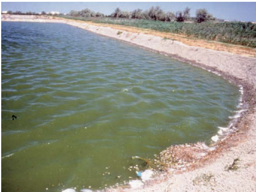
Figure 10.2 Partial view of a facultative pond in southern France treating domestic wastewater
