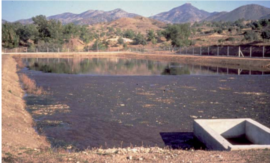
Figure 10.1 An anaerobic pond in Cyprus treating wastewater from a slaughterhouse
