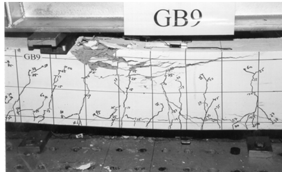
Figure 2 Deflection and cracking in FRP RC beams
