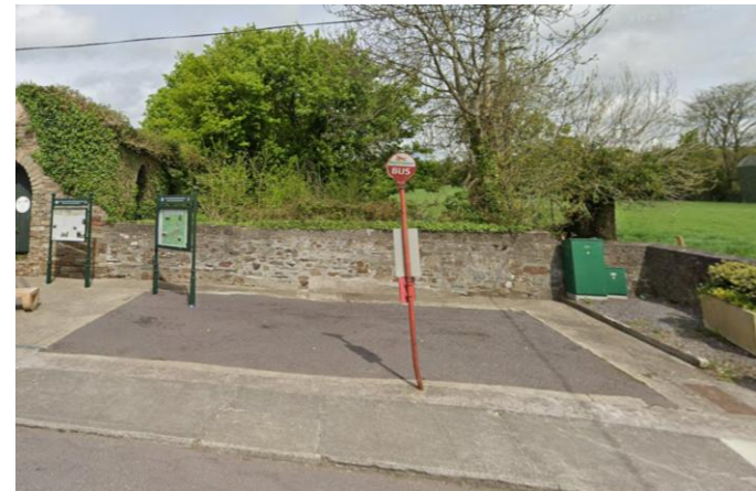
Figure 10: Site of toilets after demolition in 2021.
