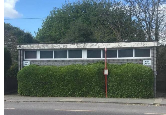
Figure 9: Original toilets from the 1970s.
