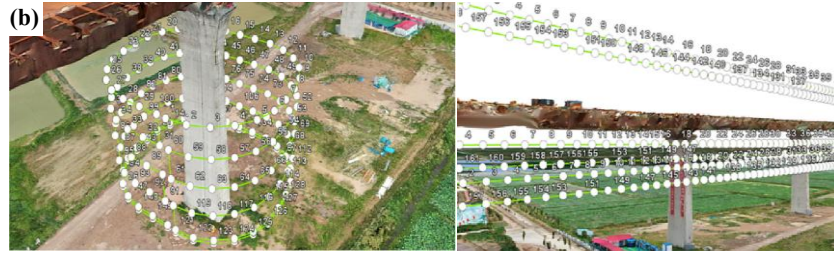
Fig. 17 a) Damage detection on railway concrete bridge [68], b) bridge 3D reconstruction [4]
