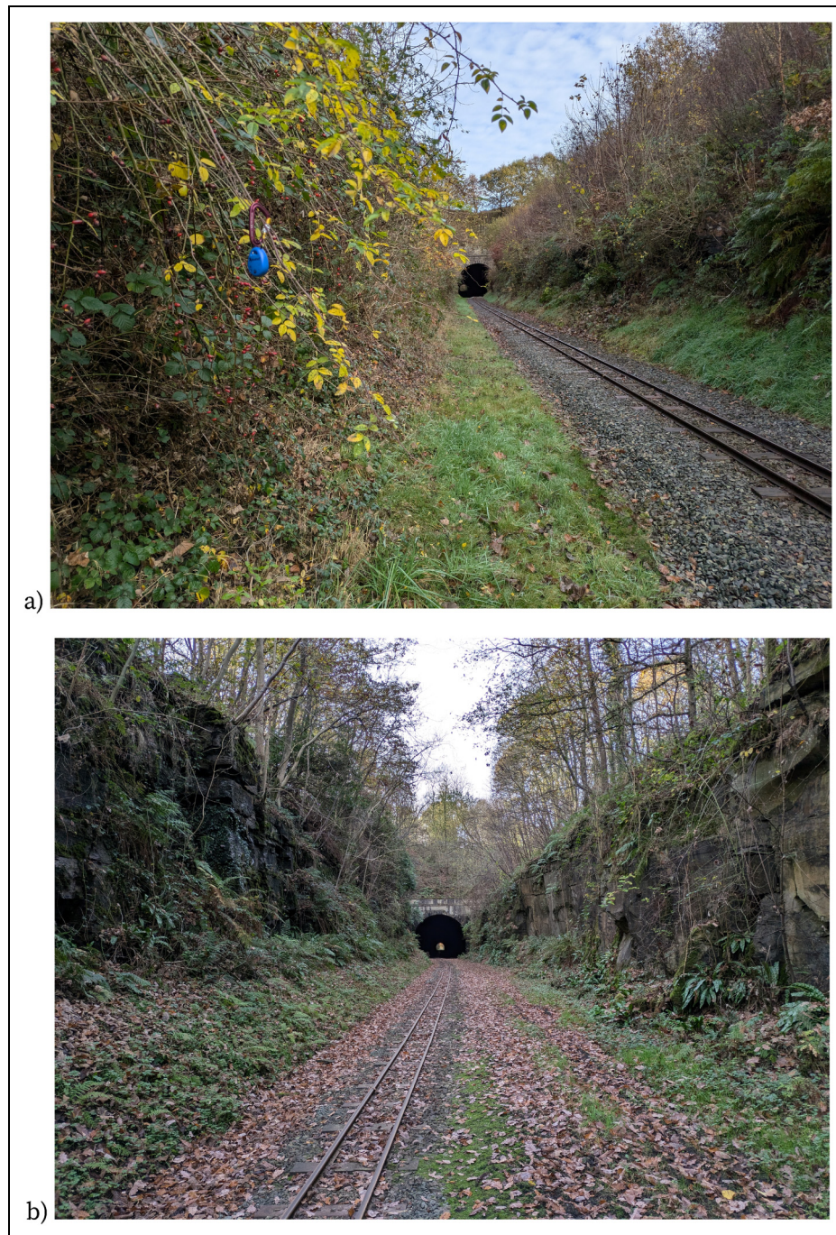
Figure 8. Cuttings at Kirklees Light Railway: (a) Shelly side (b) Skelmanthorpe side.
