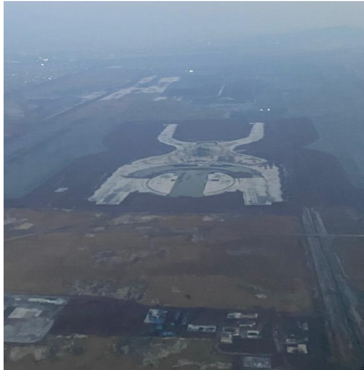
Figure 1: NAIM Layout after termination (picture taken by the authors, November 2021)
