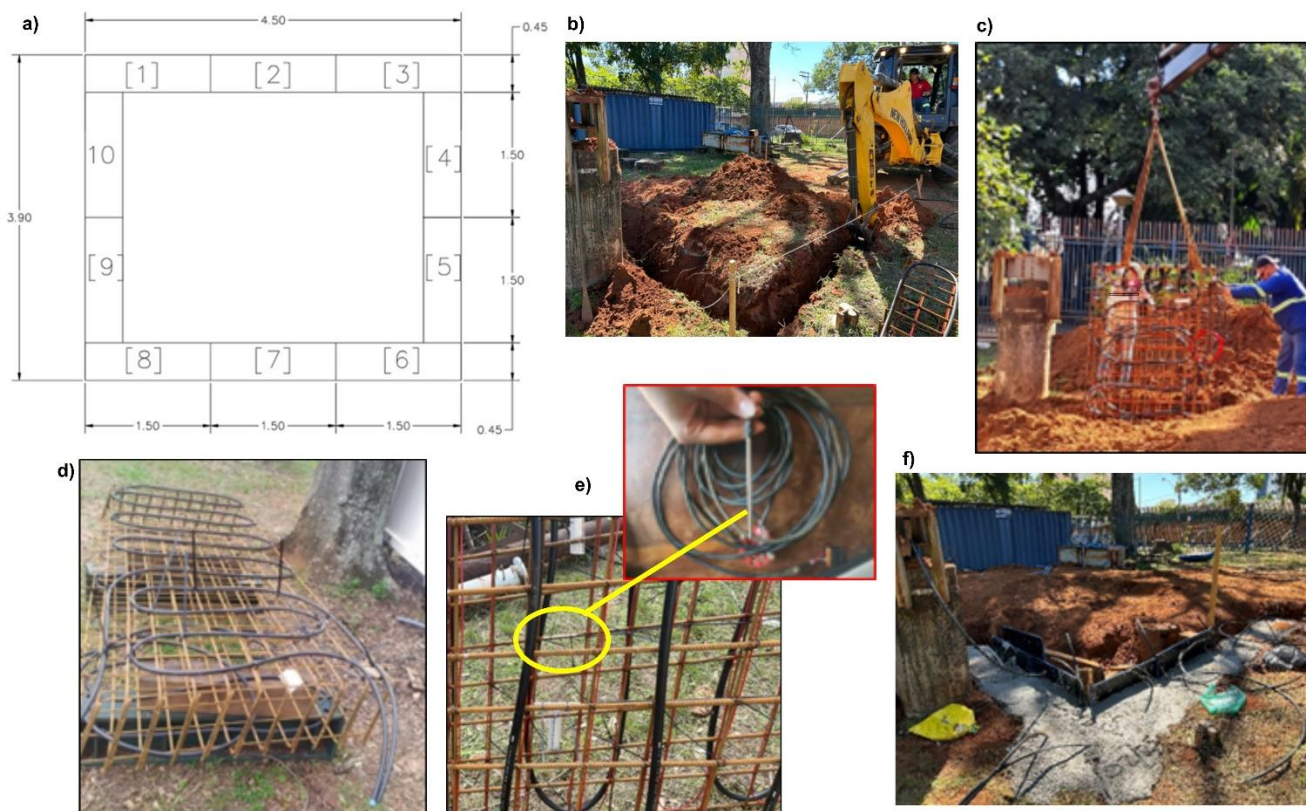
194 Figure 4. (a) Dimensions and locations of the energy wall panels; (b) Excavation process; (c) Installation of 195 steel cage with HDPE pipes; (d) Steel cage with HDPE pipes prior to installation; (e) Temperature sensors 196 embedded in the steel cage; (f) Wall panels 4 to 8 during concrete curing.
