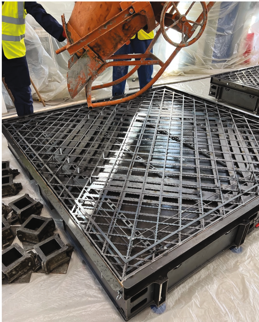
Fig. 1. Optimized LCR cage for a concrete slab.
