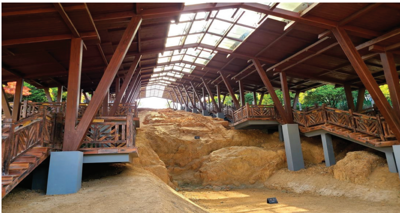
Figure 3. A typical archaeological site shelter, at Tongguan Kiln site Park, China (photo by the author, 2023).
