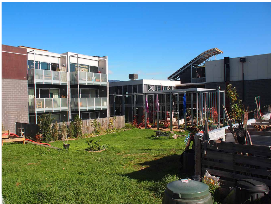
Figure 2 View of Murundaka from the back corner of garden. (Source: Matthew Daly.)
