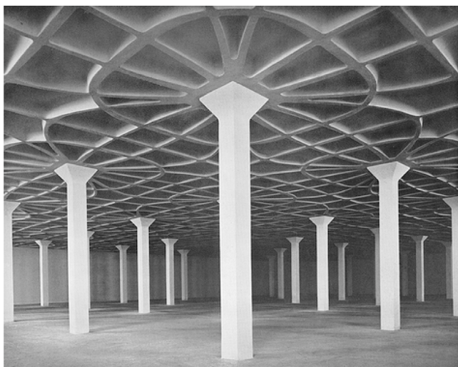
Fig. 2. Gatti Wool Factory (Rome, 1951) by Pier Luigi Nervi, showing curved downstand beams on a regular column grid [9].
