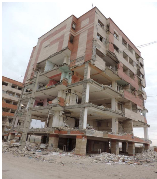
Fig. 1. Extensive damage to the non-structural components of a building after the Kermanshah 2017 earthquake, Iran (picture taken by one of the authors).
