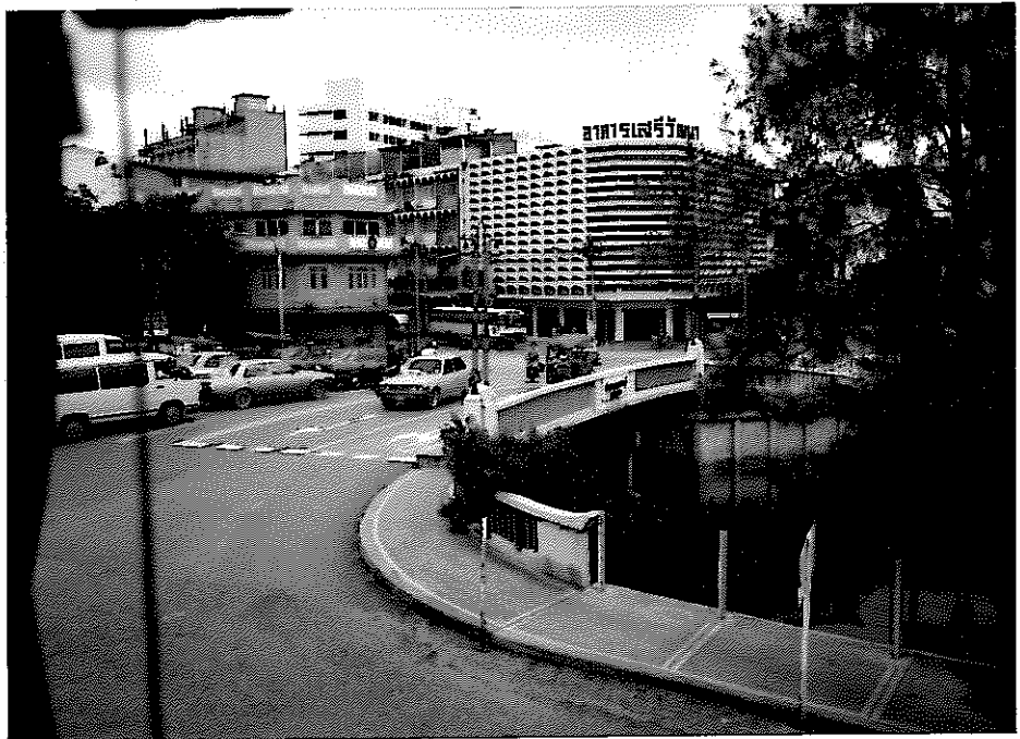
Plate 8 Junction 10 (J114) looking south-west (Stage 2 running)
