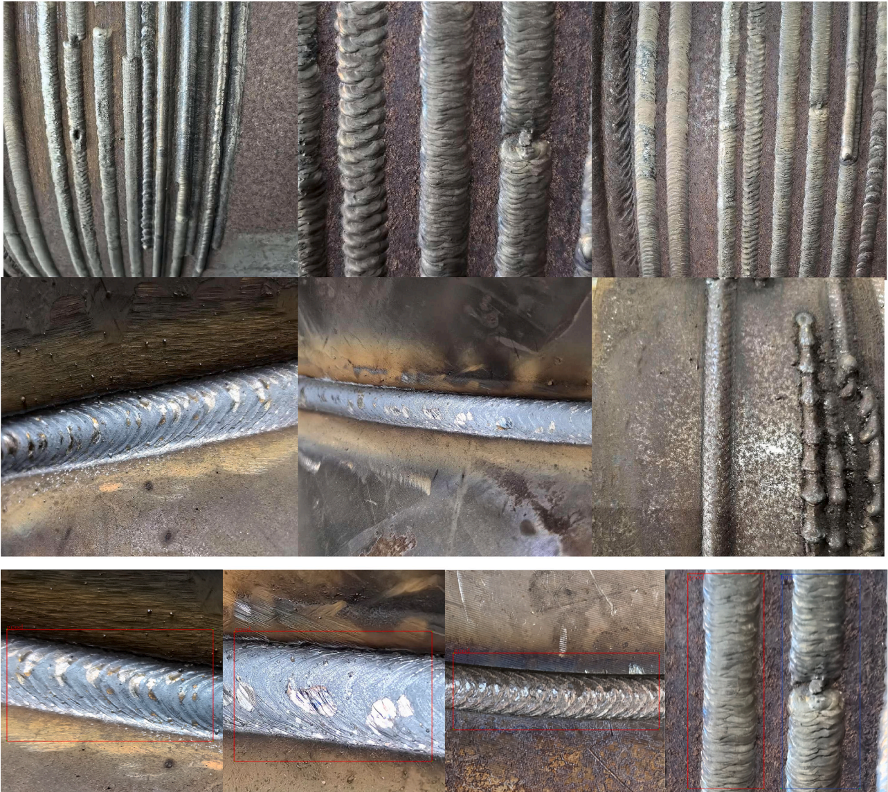
Fig. 17. Typical in-situ weld images of WAAM.
