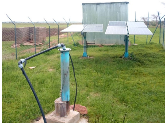
(a) Solar PV panels powering water pump
