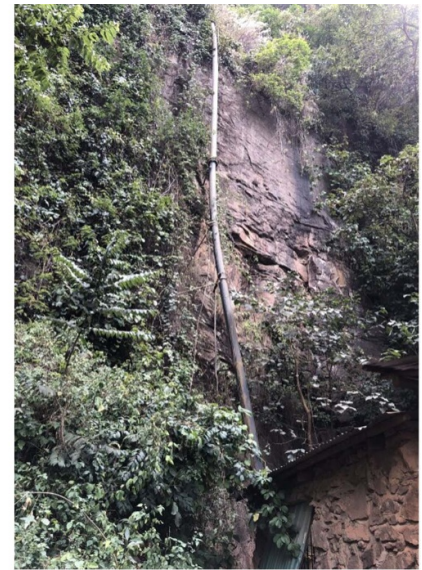
(b) Penstock carrying water to the turbine
