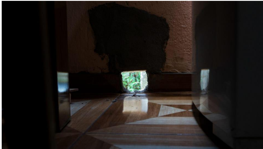
Figure 1. Picture of a hole in the wall opened by a dweller during a flood (and kept open for precaution). Source: Lucas Lourenço (2021).
