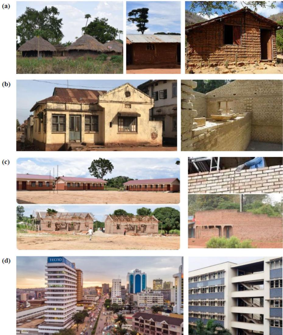
**Fig. 6** Common building types constituting Uganda’s building stock: **a** wattle-and-daub, **b** adobe with mud mortar, **c** fired bricks with cement mortar, and **d** modern-style buildings
