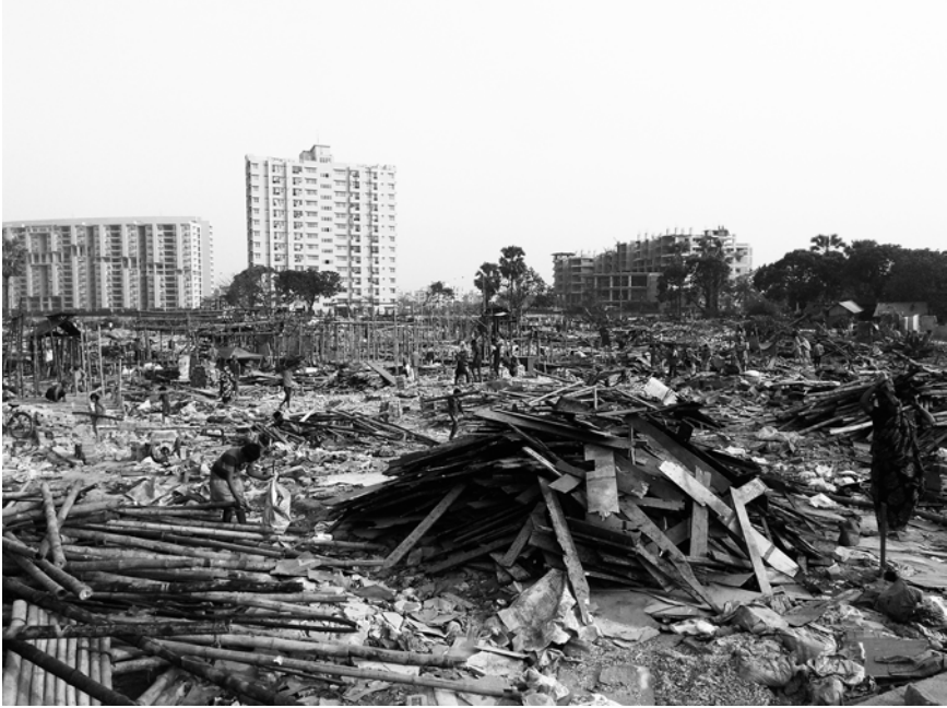
Figure 7 The aftermath of a recent eviction at Bhashantek settlement, Dhaka, 2019. (I arrived just a few hours after it was bulldozed to the ground.)
