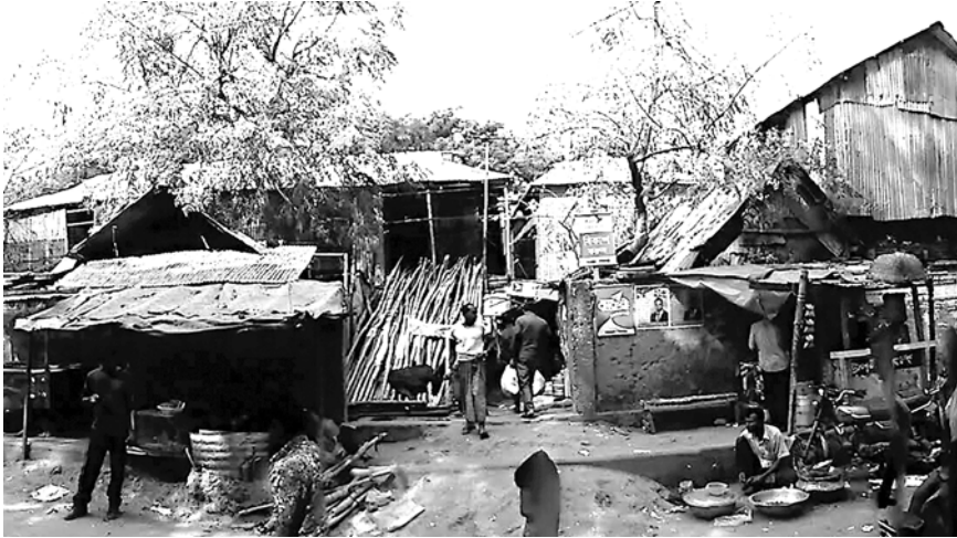
Figure 5 How the newly built wall in 2013 was overtaken (and almost hidden) by 2019. (Structures are built over the boundary wall, engulfing it and obscuring its view from the street.)
