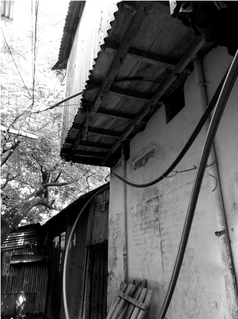
Figure 10 A house built on top of the 'community' public toilet that is no longer public.
