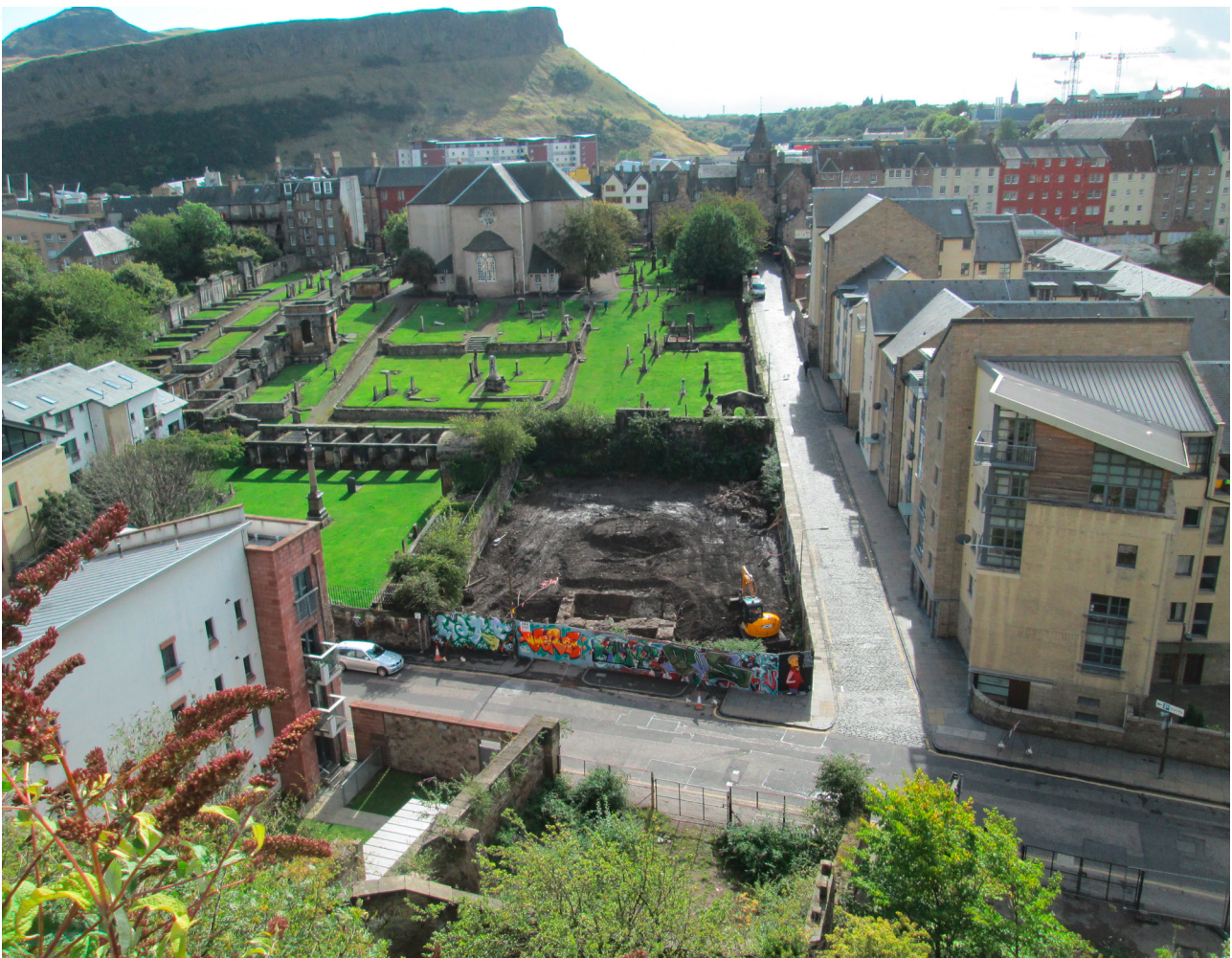
Illus 1 South-facing view of the New Waverley site under excavation, showing the relationship with the Canongate Kirk and Kirkyard
