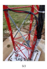
**Figure 1.** (a) Photograph of the LUMO structure, (b) A schematic of the structure highlighting measurement levels (ML) and damage locations (DAM) with the reference axes, and (c) Damage location 6 (DAM6) displaying the reversible damage mechanisms. Images reconstructed from Wernitz et al. (2022).
