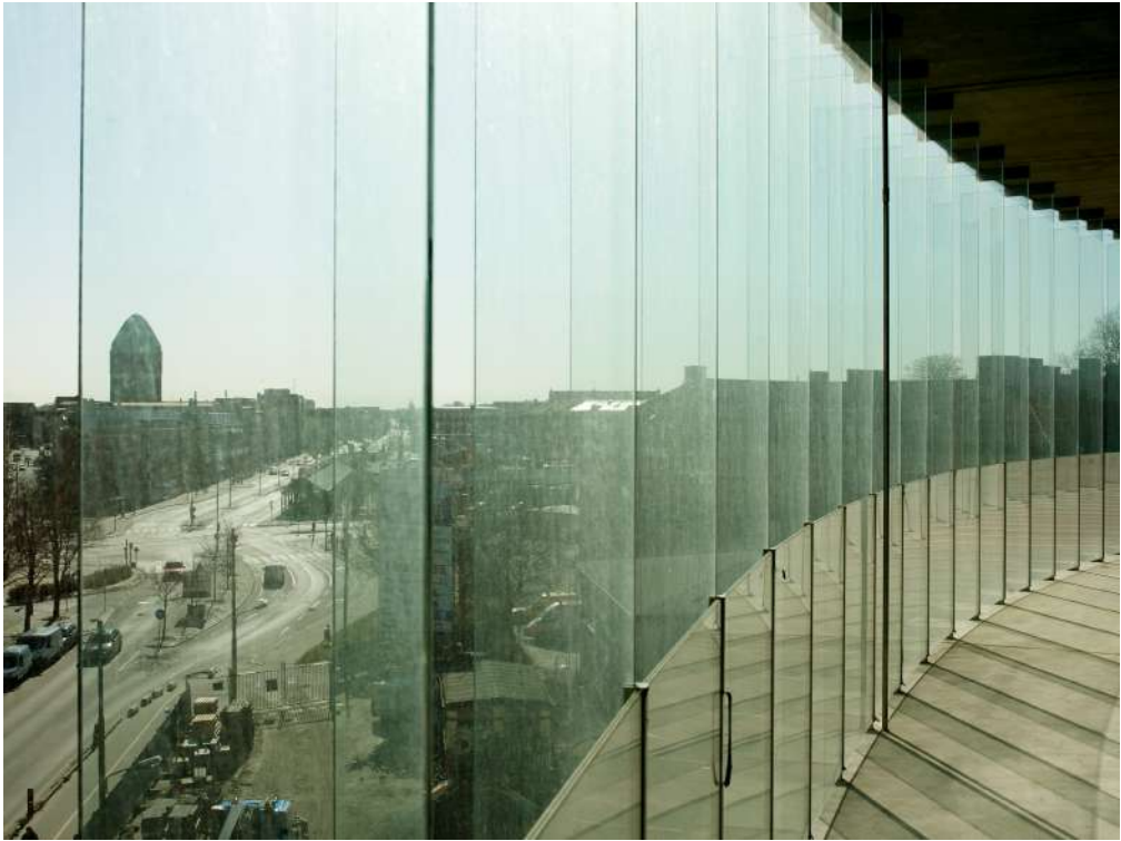
Figure 4: Glass Lamellae at angles to allow natural ventilation (Source: C.F. Møller Architects + Jørgen True)
