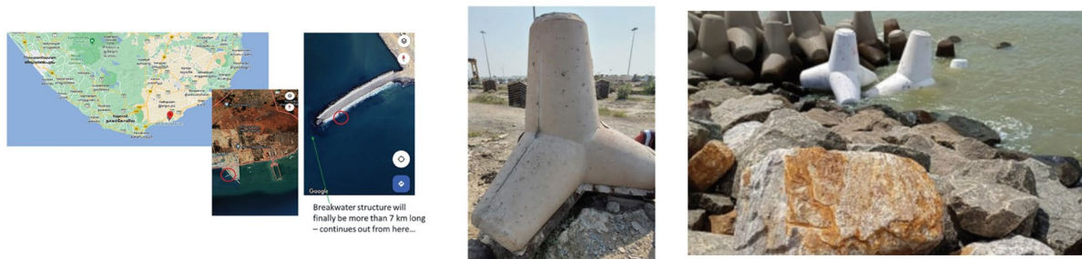
(B) Tetrapod produced LC2 admixture replacing 30 % of PPC cement [252]
