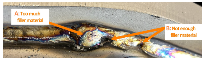
Figure 2: Typical welding issue where there is buildup of filler material (A) and coverage is not sufficient (B), creating an irregular and weakened weld.
