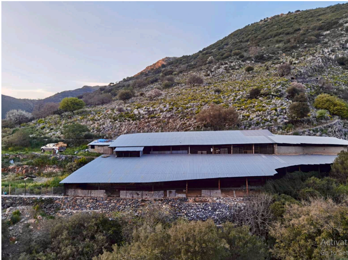
Photo 2 Livestock Housing Unit, Case 4, photo supplied by farmer.
