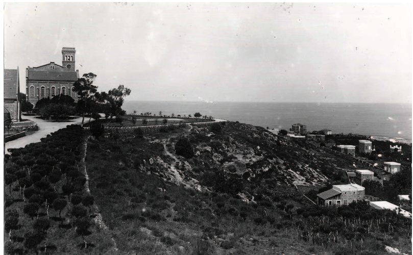
Figure 2 Main Building (College Hall), Syrian Protestant College, Beirut, 1873, view from the east in the 1890s (Moore Collection, Library Archives, American University of Beirut).
