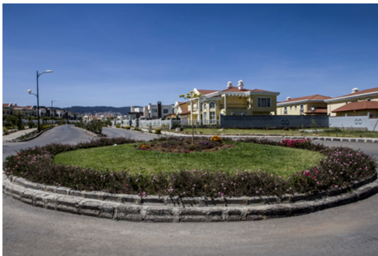
Figure 9.1 Country Club Developers, Legetafo, Addis Ababa (source: Mark Lewis)
