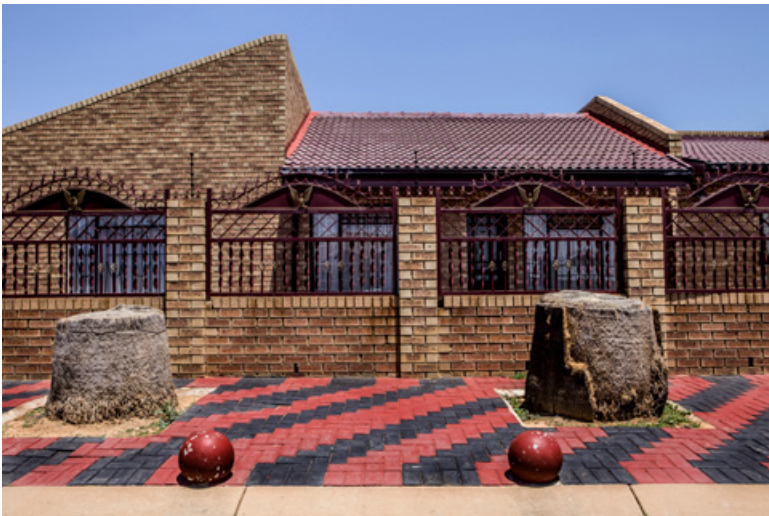
Figure 6.3 Housing improvements in Ekangala (source: Mark Lewis)
