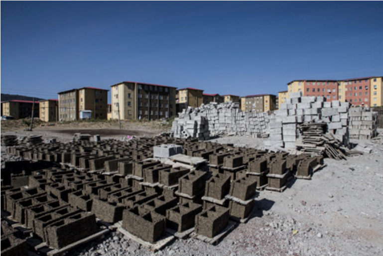
Figure 5.1 Construction materials and condominium housing in Yeka Abado (source: Mark Lewis)
