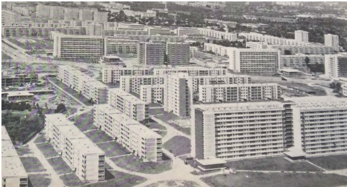
Figure 5. Balta Albă Housing District, Bucharest, Romania, 1967. Image published in Arhitectura , no. 4 (1967): 31. (C) Revista Arhitectura , Bucharest.
