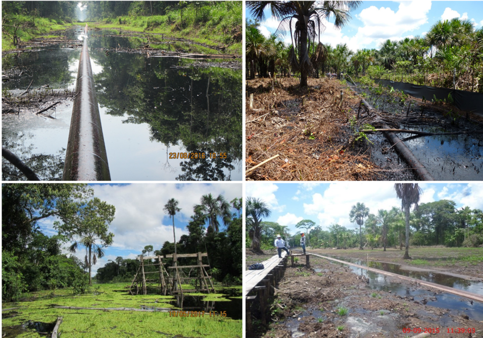
Figure 5. Oil infrastructure and contamination in the wetlands and peatlands of the Pastaza-Marañón Basin in Peru. Top left: dredged channel showing an oil pipeline during low river level. Bottom left: an oil spill at Lot 8 inside the Pacaya Samiria Nature Reserve, 2013. Right: remediation of a November 2014 oil spill near Cuninico showing the clearance of peatland vegetation during periods of (top) high and (bottom) low river levels. Source: All OSINFOR (InfraAmazonia 2021) except bottom left, ACODECOSPAT (2019).
