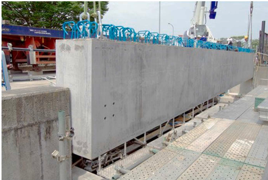
Fig. 1. In-service example of a 150 MPa Zero Cement Concrete element being used to construct a bridge [14]. The material depicted, marketed as "Sustain-Crete", is a commercial product resulting from the lines of research and development described in this article and using the same mix design principles.
