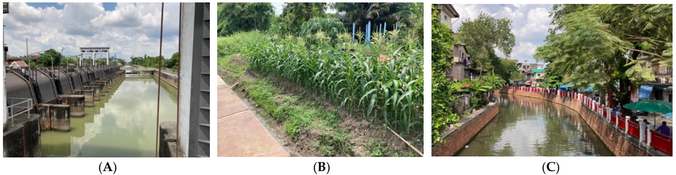
Figure 5. Pumps at the watergate in Saneab Canal (A); edible plantation (B); renovation of the embankment by historical material in Banglampoo Canal (C).
