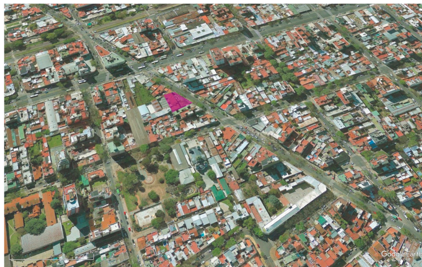
Figure 2. Aerial view of the Medone school neighbourhood context with the school ground in purple highlight. Source: Authors' own image based on data from Google Earth. Available online at: https://earth.google.com/web/ (accessed on 1 August 2024).
