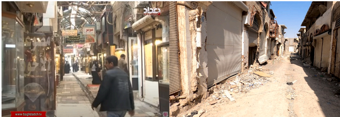
Fig. 15. Souq Al-Sayagh as seen in a video from 2013 (left) and September 2020 (right).
