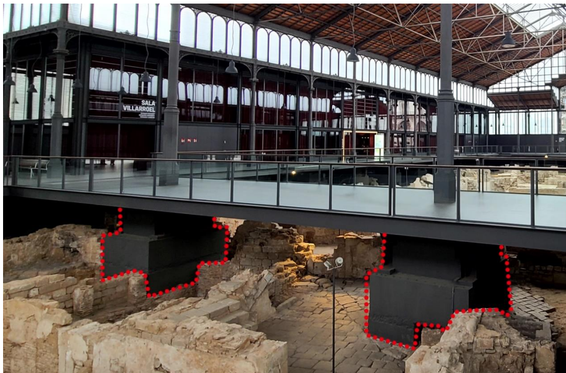
Figure 3 The inevitable overlap between the museum building foundations and the site (El Born Centre de Cultura i Memòria)
